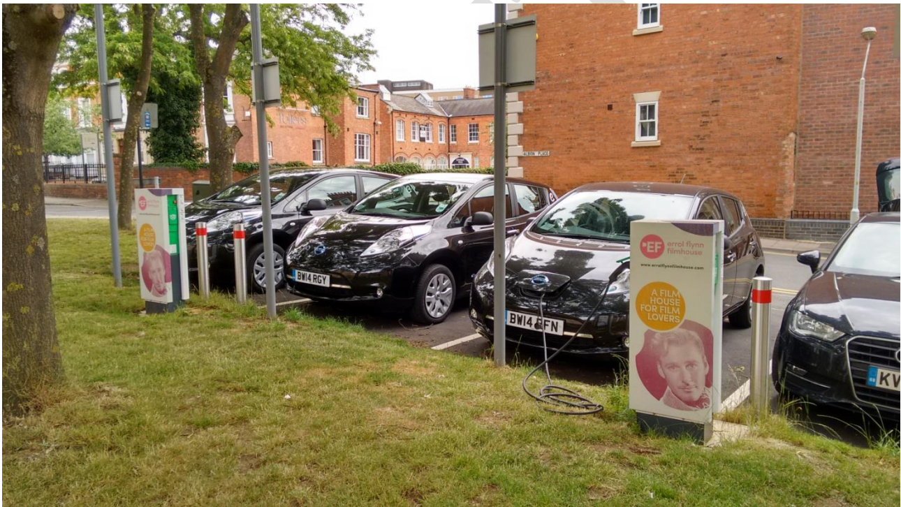
Figure 7 – Northampton EV Recharging
